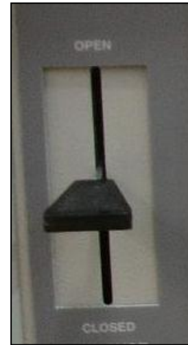
Figure 4. Damper Positions.
